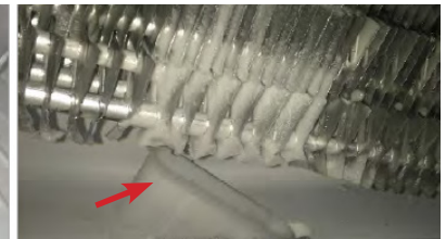
Remove Drain Ferrule
